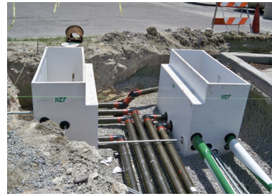
Twin Sumps House Transitions
