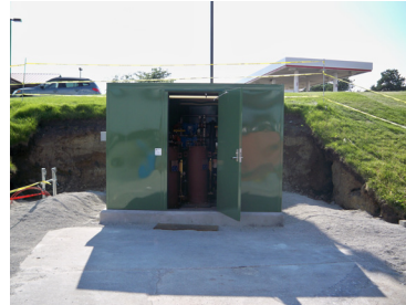
Pre-Fab Building Installed Over Sumps and Blend Fixture
