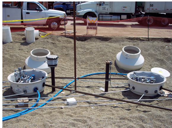
2 Sump Mounted Blenders
